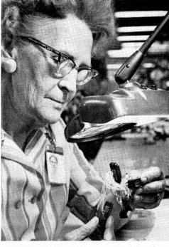
WIRING HARNESS is assembled by Mary Kelley. In addition to making cables, the Section assembles printed circuit boards and fabricates wire harnesses for junction boxes. The work is usually one-of-a-kind prototype assembly and requires painstaking care.
